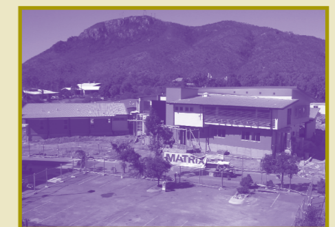
The Palliative Care Centre - under construction
